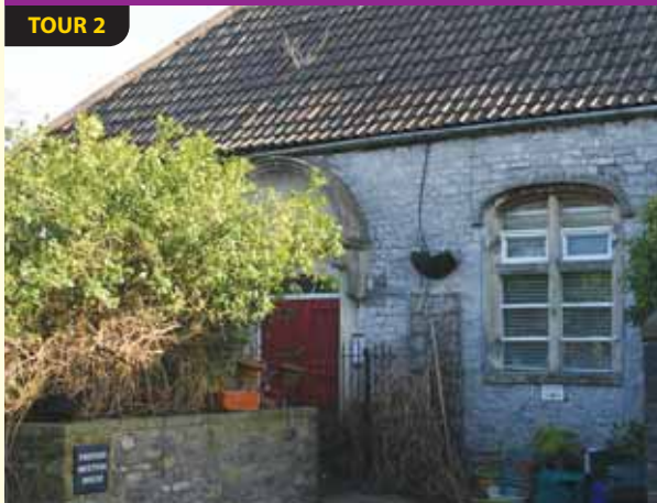
Chipping Sodbury, Friends Meeting House
