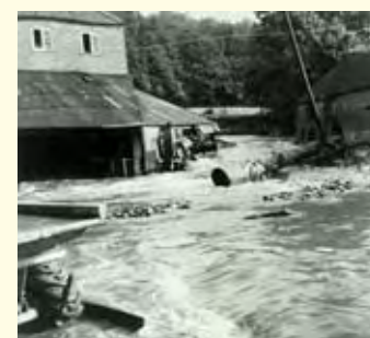
Scene in front of Willsbridge Mill July 1968 after breaching of Dam wall
